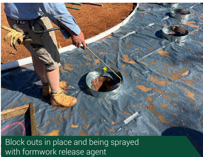
Rectangular and round block outs in place ready for concrete pour
