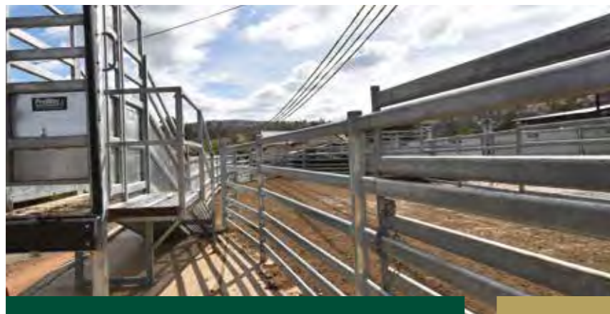
Look up and live. Overhead power-lines are a serious danger throughout the construction of your yards.
