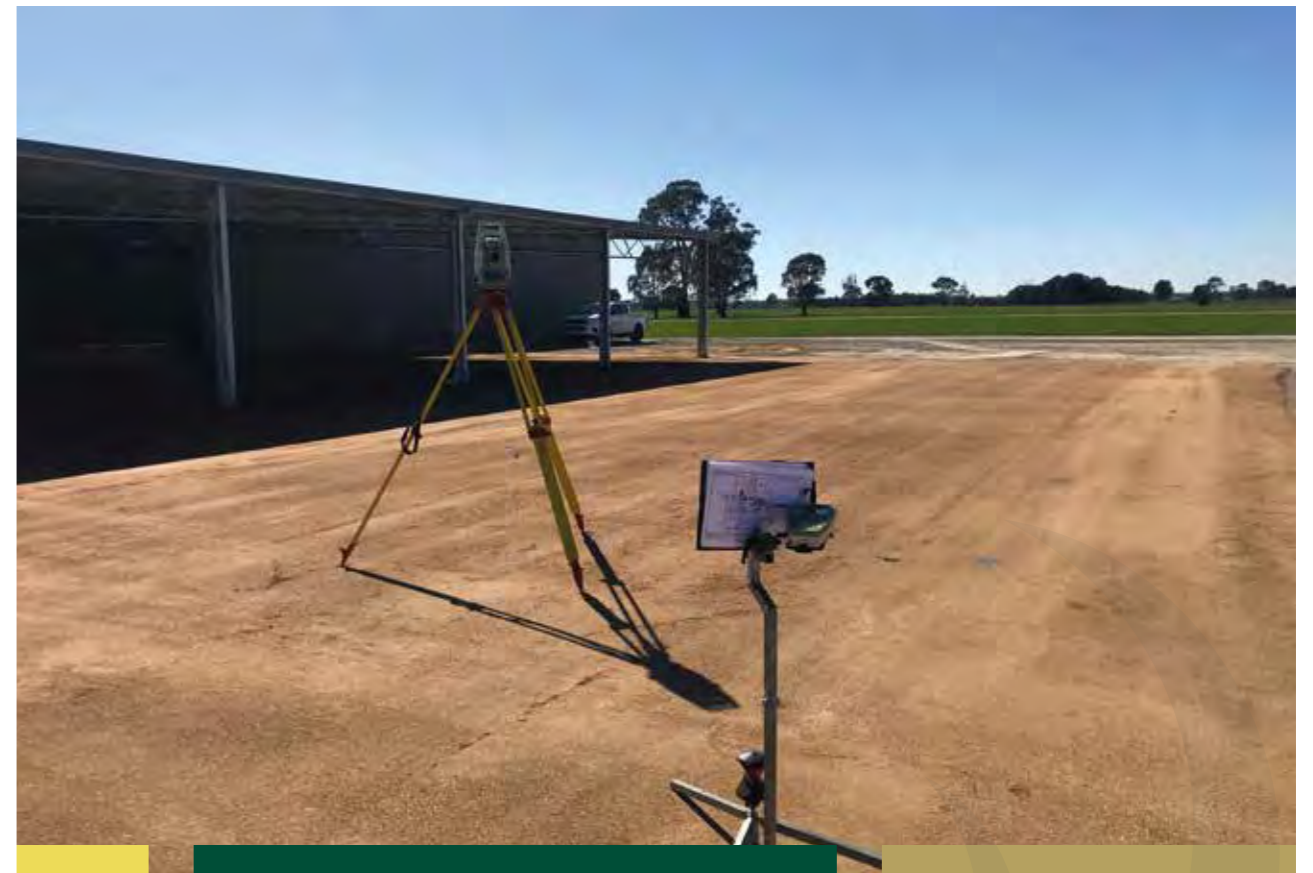
A combination of measuring tapes and survey equipment is used to peg out the yards accurately and efficiently.
