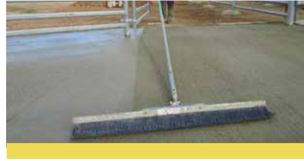
Slabs have a broom finish for human and sheep traffic areas.
