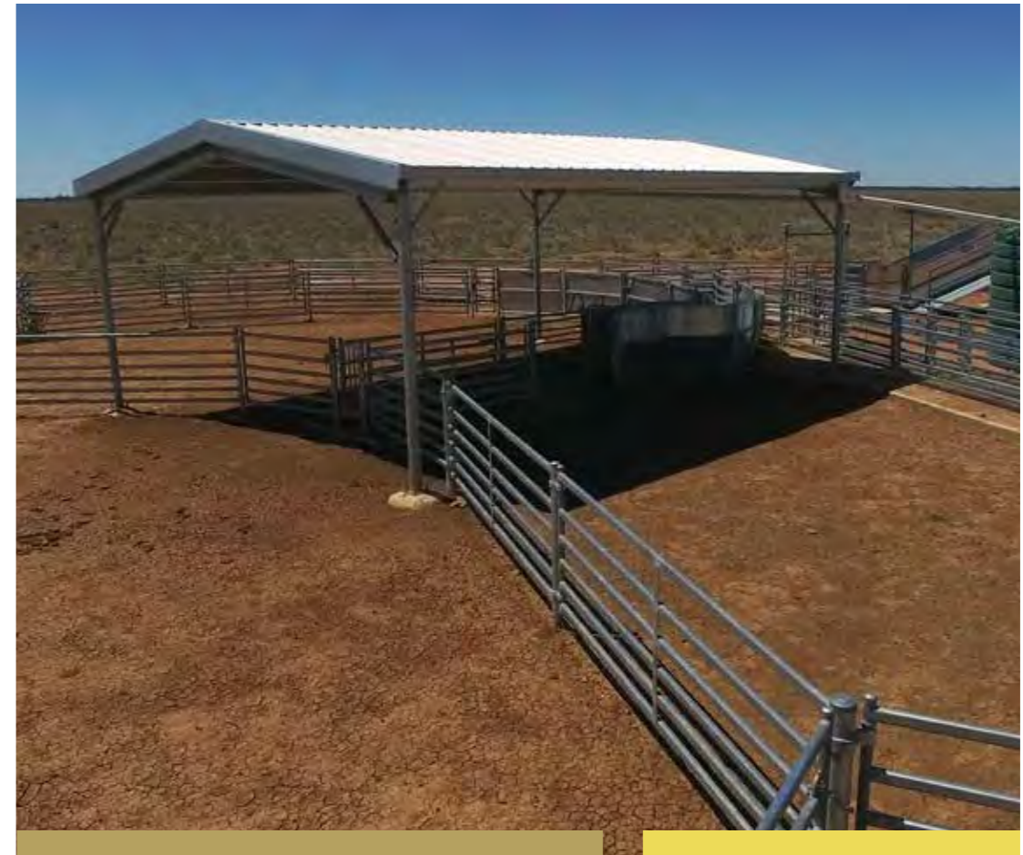
If you have a roof, consider the runoff and how you can use the water effectively.
